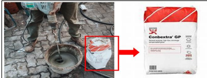
Figure 2. Grout Mixing Preparation using Fosroc Conbextra
