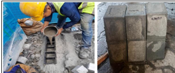
Figure 3. Cube molding and Demolding
