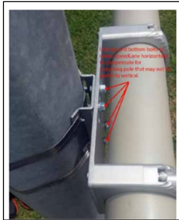
Figure 6. Installation of the mounting bracket (Houston Radar, 2018).
